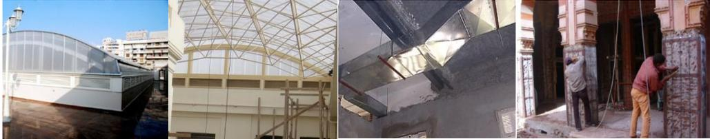
Fig. 3: (Left to right) metal truss for roofing the central area, air conditioning network, and supporting the arches in the central area of the ground floor (curtsey to Culture Development Fund).
