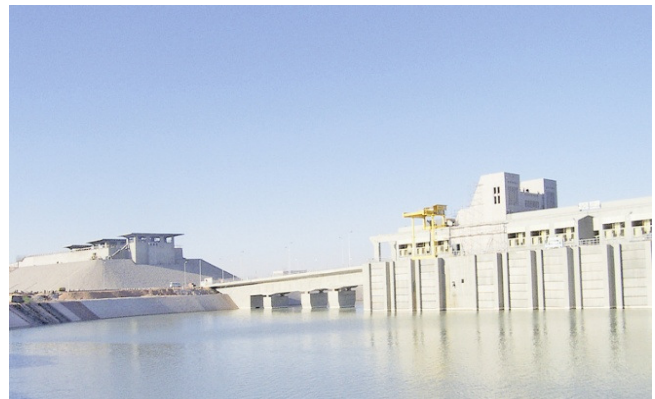
Fig. 1. Toshka Pumping Station
